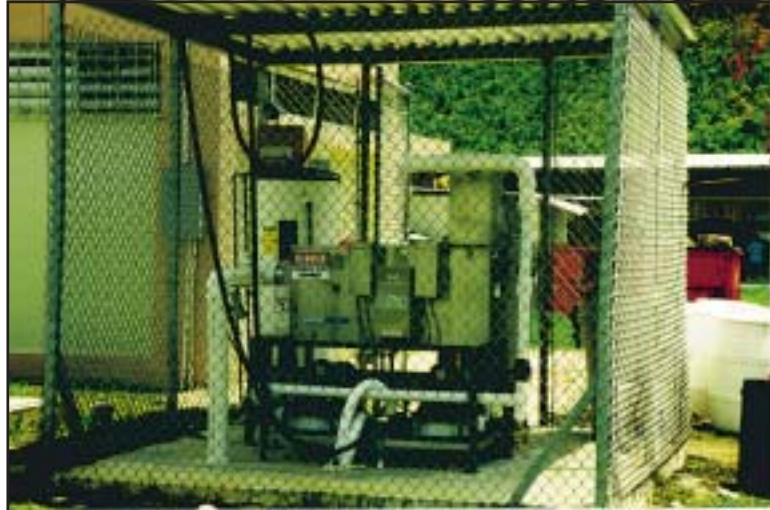
Pictured is one of two Big Dipper® SuperCeptor® grease/water separator systems located at the Sabana Hoyos Correction Institution and Sabana Penal Camp in Puerto Rico. The units are in an outdoor location for pretreatment of kitchen water.
